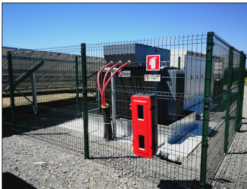
Plate 3-14. Typical transformer compound fencing
