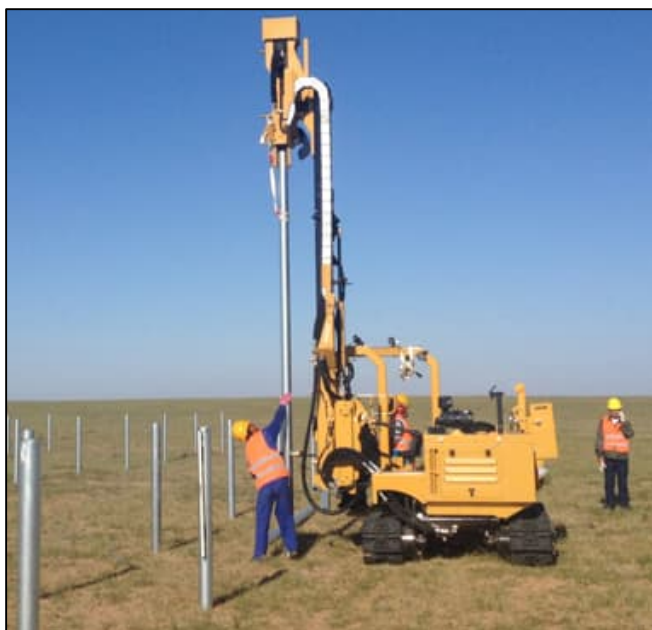
Plate 3-18. Ramming of module mounting structures.
