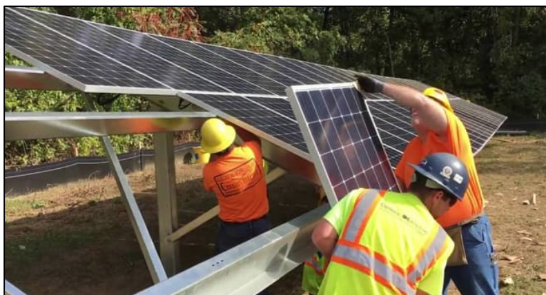
Plate 3-19. Construction staff mounting solar PV modules by hand.
