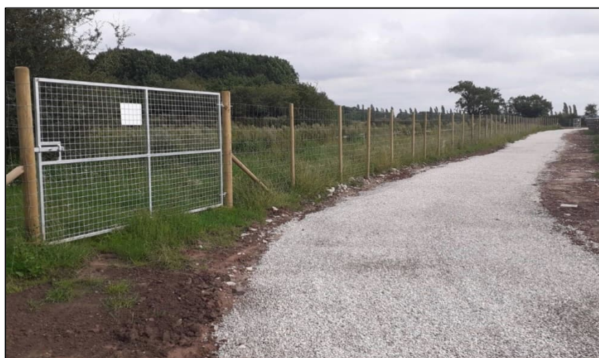
Plate 3-17. Example of an access path.
